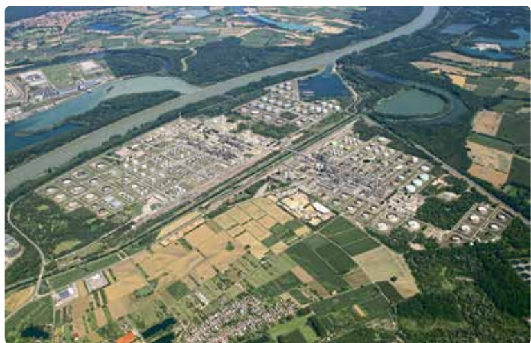
Oberrhein mineral oil refinery (Miro) is the largest German refinery.
