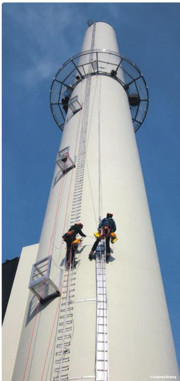
The new exhaust air extraction system: one of the two new exhaust chimneys with emission measuring points on the 43-meter-high working platform.
